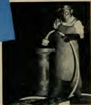
• Weld inspection by Gamma-Ray Radiography—modern technique in use at Todd yards—records internal cracks or cavities on film.
